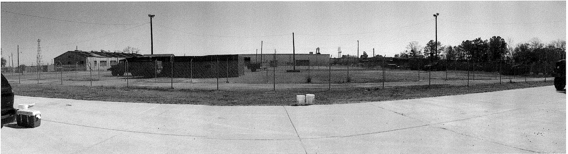
View South From MW-1
