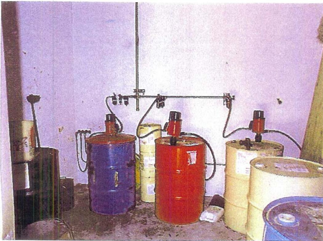
Photo 2. POL Storage for air operated machinery.
