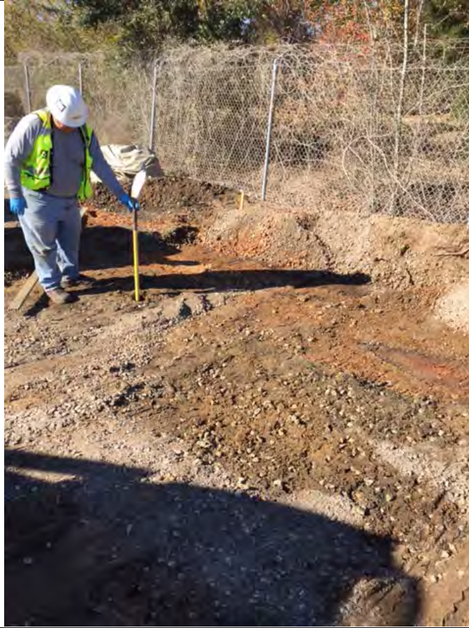
Photo 11 of 12 - Borehole where OMS-28-6 once existed.
