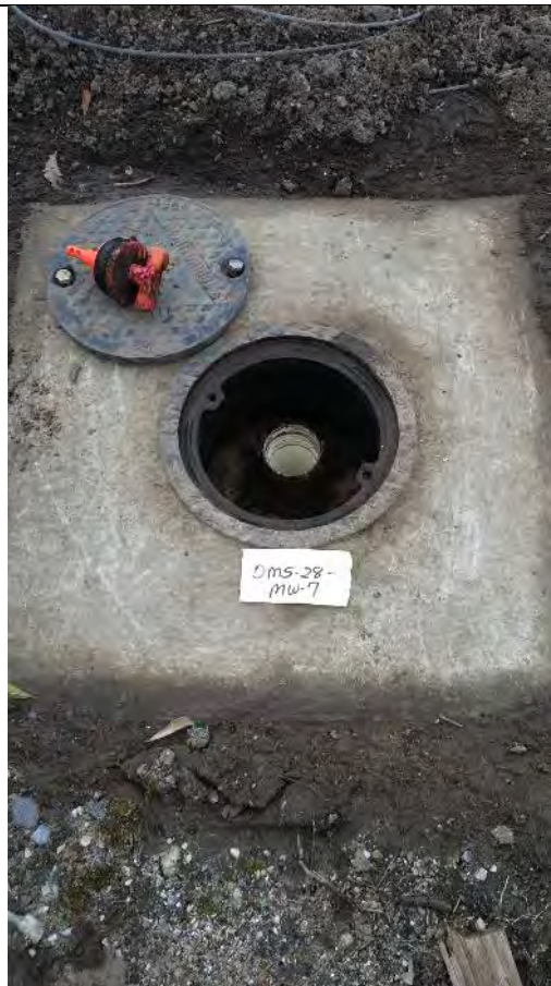
Photo 12 of 12 – Condition of well OMS-28-7
