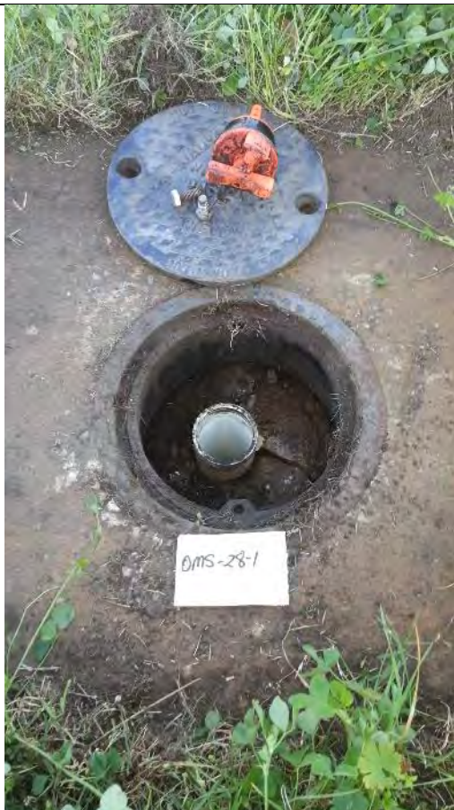
Photo 6 of 12 – Condition of well OMS-28-1.
