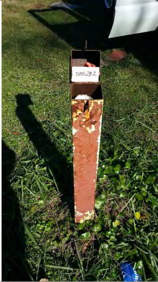
Photo 7 of 12 – Condition of well OMS-28-2
